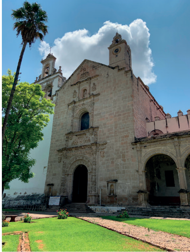
fig. 5. Cuitzeo, Michoacán, Mexico, St. Mary Magdalene, Augustinian monastery (construction began in 1550). Photo by Juan Luis Burke.
