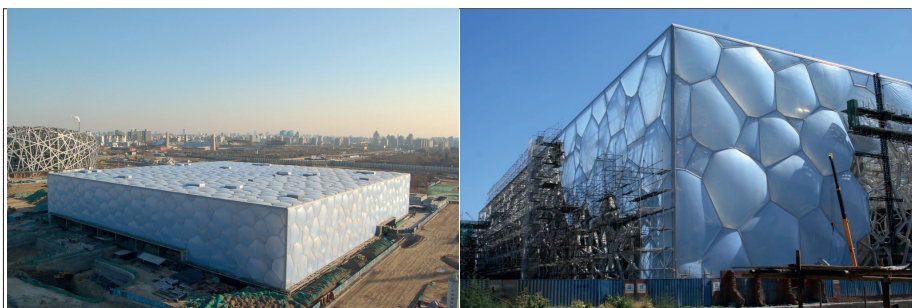
Fig. 2.1 e Fig. 2.2. Aerial view of the Water Cube and detail of the ETFE-clad structure (Wikipedia.com)
