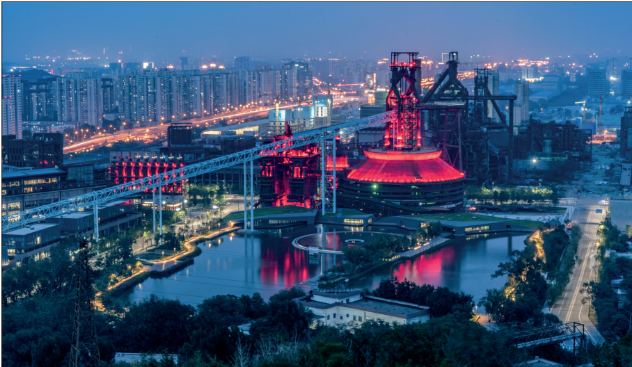
Fig. 10. View of the blast furnace from the west side (Photo ©Zhujing Design)
