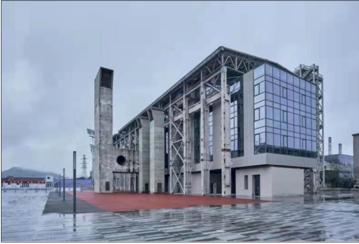
Figure 9. Big Air venue in Shougang Industrial Park, Visitor Center within the former Oxygen Factory designed by Politecnico di Torino. Source: G. Cestaro, 2022
