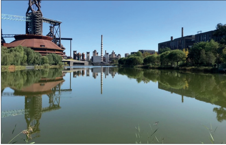
Figure 10: Qunming Lake (cooling pool) in Shougang Industrial Park Source: G. Cestaro, 2022
