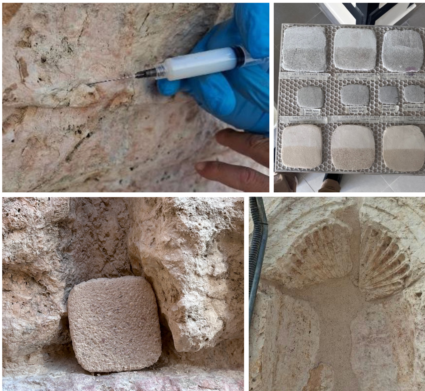
above, from left, Fig. 18 Re-adhesion of flakes.
