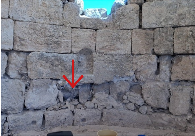
Fig. 23 Sample 9. General view, in the middle of the wall.
